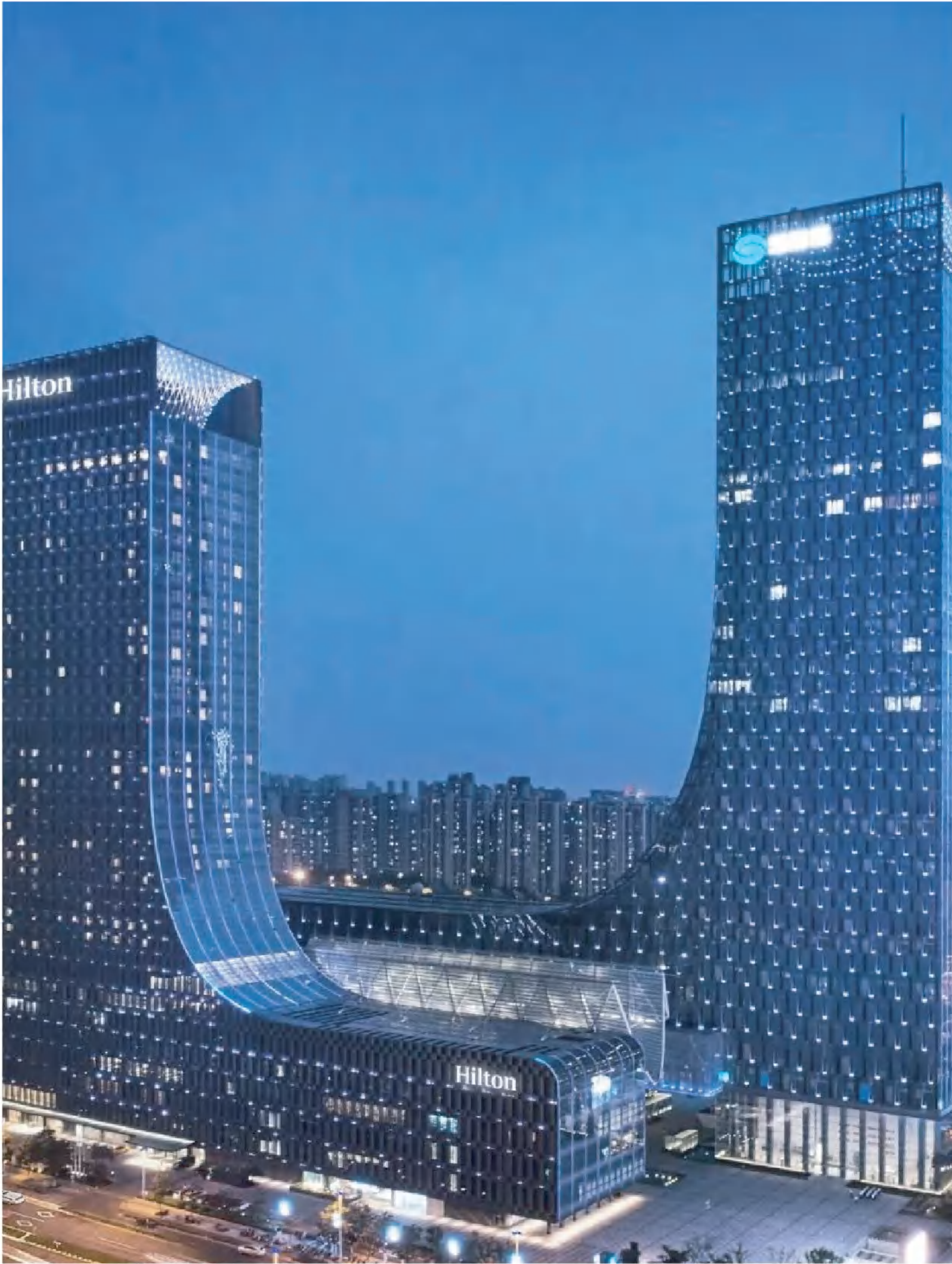
SUZHOU-SUZHOU Radio And Television Station Construction Areas: 60000 square Meters Product Series: OA600 Steel Access Floor Panel 工程名称: 苏州·苏州广播电视台 工程面积: 60000平方米 产品系列: OA600钢质网络活动地板
