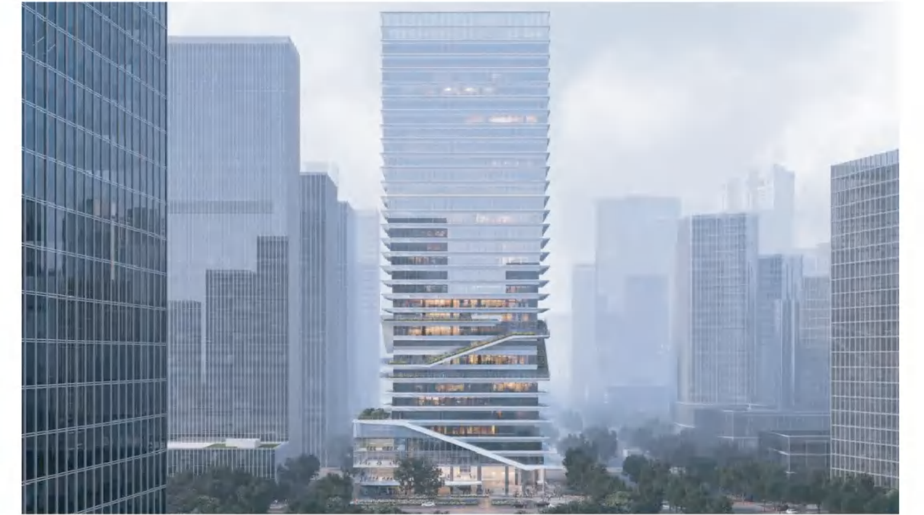
SHENZHEN-ByteDance Houhai Center Construction Areas: 100000 Square Meters Product Series: OA600 Steel Access Floor Panel
